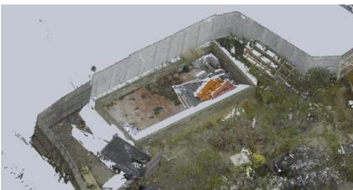
A close up of the foundations from a previous building in the harbour, which EAPL used as the basis for their new building.
